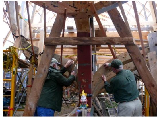
Roy Jenkins drills out the first futtock for the permanent trunnels then drives home the trunnel. then The lag bolt used to keep the frame fair between fitting and trunnelling is then removed.
