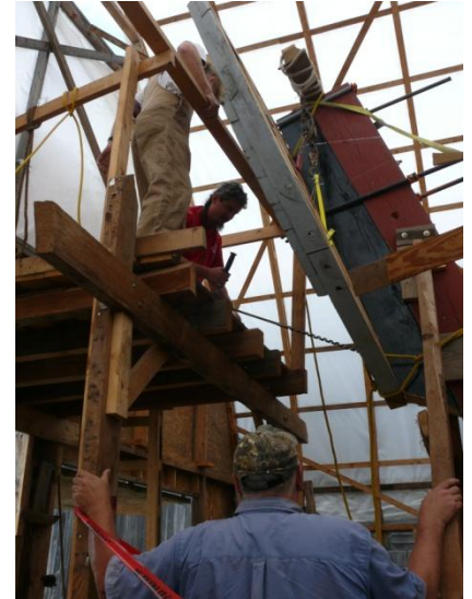
Jeremy and Tim work the 3 foot drill from the work platform.
