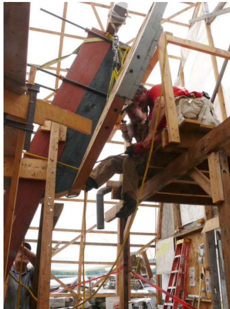
Jeremy and Tim work the 3 foot drill from the work platform.
