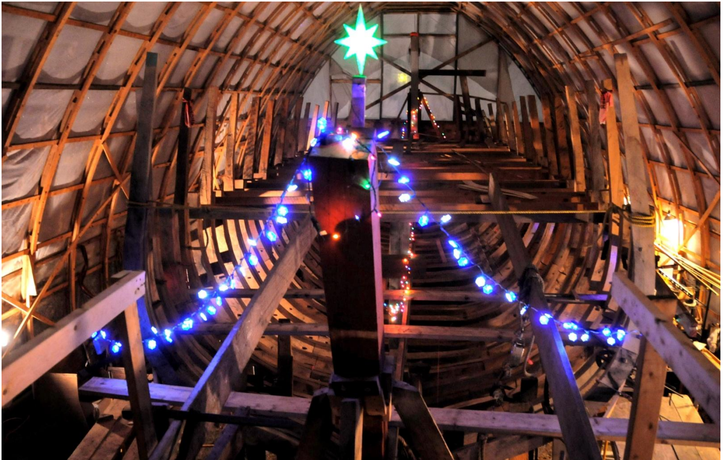
Professional photographer Paul Cunningham view of Virginia from the high rise work platform constructed at Virginia's stern
