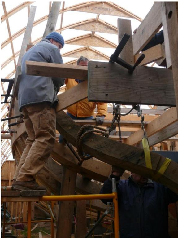
Each frame is fitted snugly into the preserved mortise and then "tuned" in 3 dimensions.
