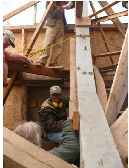
Below, Orman and Tim Teague discuss the angle measurement of the stem rabbet and how it fairs into the knightheads in preparation to receive the planking
