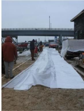
roof material was laid out and attached to stabilizing strapping. Ropes were tossed over the boatshed frames at intervals and on the signal volunteers hauled away! A brief snag cleared with a gust of chill breeze and the new roof was quickly in position and being secured by strapping and screws, on both sides of the
