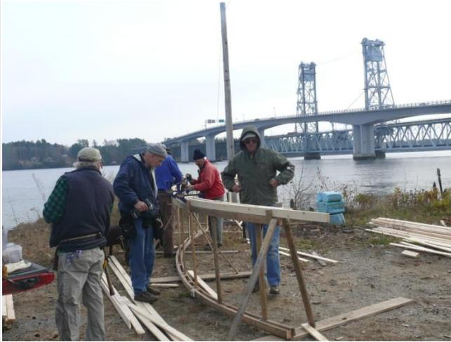
were salvaged, repaired and stabilized into a vertical jig. Twenty one boatshed frames (consisting of 42 halves) were fabricated. New frames were built on top and parallel to the old using West Systems epoxy and screws. This jig design was a great improvement over the horizontal jig, allowing many volunteers to work together on each frame, bending, clamping, applying epoxy and screws. The crew became so proficient over time they were able to turn out a new frame in 30
