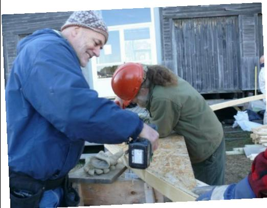
Gussets were used to join the two halves and each frame was raised and attached to the knee wall.
