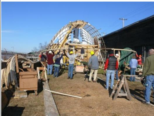
As each frame was raised it was attached to the ridgepole and horizontal stiffeners were added and then diagonals to create a structure strong enough to last
