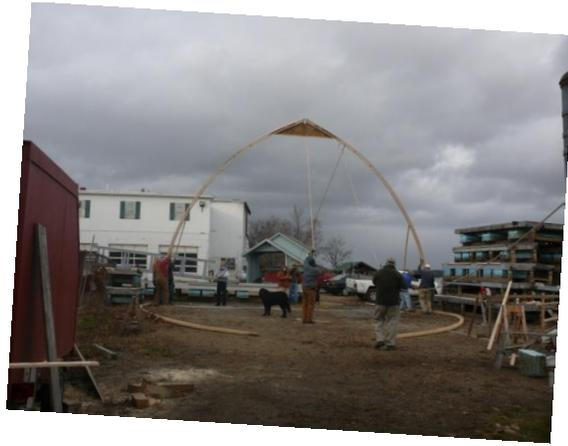
After standing up each frame, carry poles and guide ropes were used to “walk” each end of the frame across the gravel lot and around each side of the boatshed.
