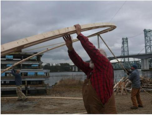
**Rebuilding the boatshed:** Raising the last 6 frames. Although the original damage evaluations indicated the last 6 boatshed frames could be salvaged, they looked “so bad” in comparison to the new frames, volunteers demanded they also be replaced. The last 6 frames were raised over the partial north rear wall of the boatshed.
