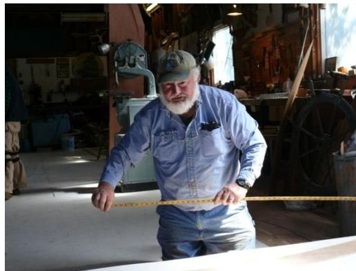
Orman Hines on *Virginia's* lofting floor this winter, measuring offsets, a series of plotted points from the ship's drawings that are "offset" from a specific baseline in the drawing. Offsets are used to increase the scale size drawing into the full size pattern. Orman has been active in *Virginia's* construction and teaches history to the RSU#1 Summer Shipbuilding Program students.
